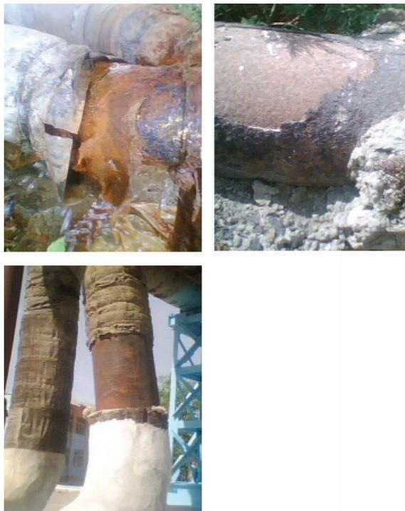
**Figure 1:** Typical corrosion in long-term use of basaltic-fibrous materials for insulation.
