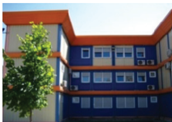
Figure 2: Case study: Intermodal steel building units used for office purposes.
