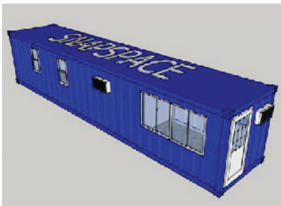
Figure 1: Intermodal steel building unit (ISBU).
