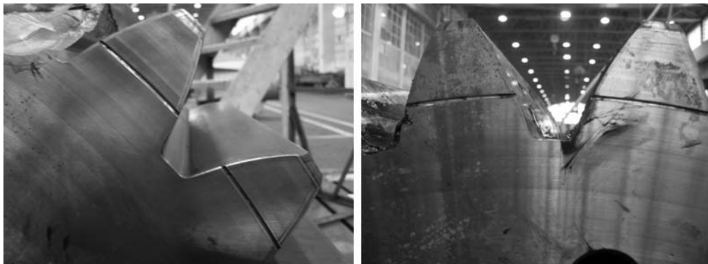
Figure 2. A broken tooth and two unbroken teeth with a fatigue crack (left). Two failed teeth: the lines indicating the heated surface (right).
