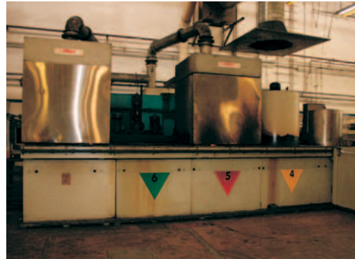
Figure 6. System for heat treatment after installation of the second device.
