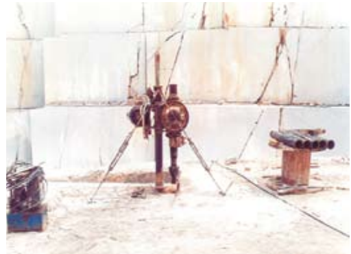
Figure 4. Drilling of vertical bores using a drilling machine
